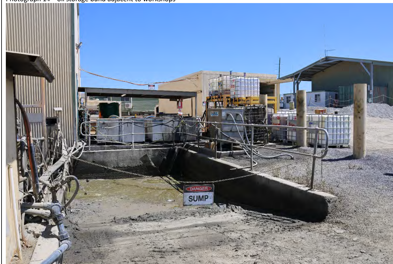
Photograph 15 – Oily water collection sump behind heavy plant maintenance workshop
